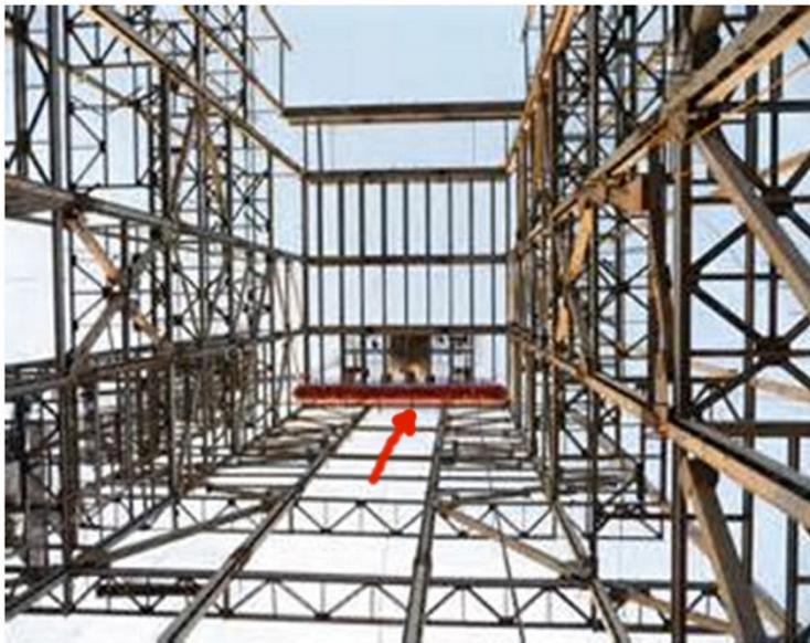
Figure 9.1 – Typical Steam Drum Installation
